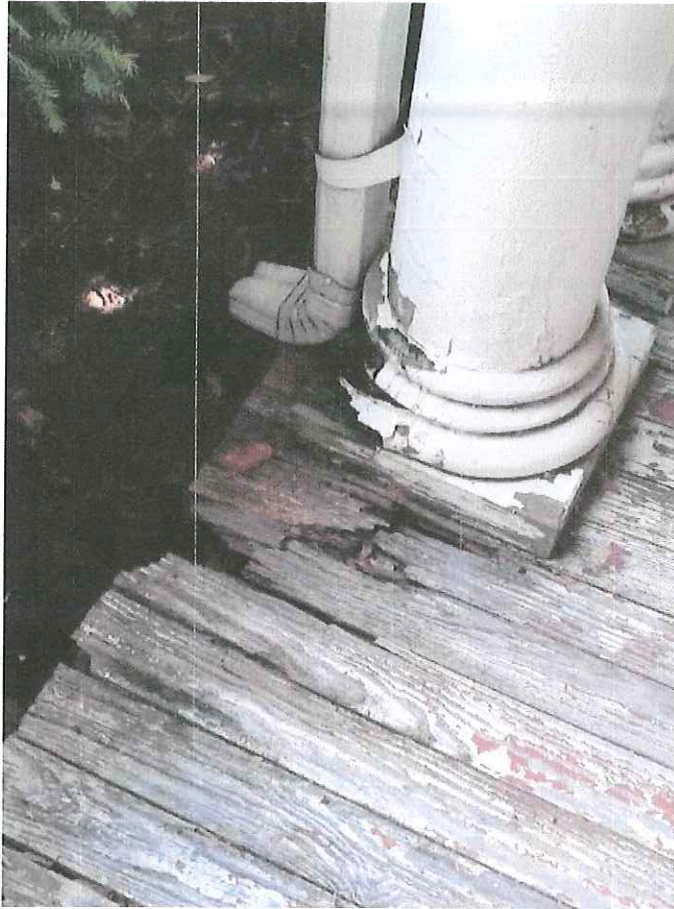
Photograph #4 – Porch floor and supporting columns
