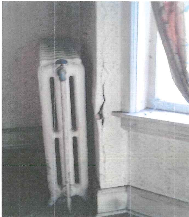
Photograph #8 – Interior bay window sills
