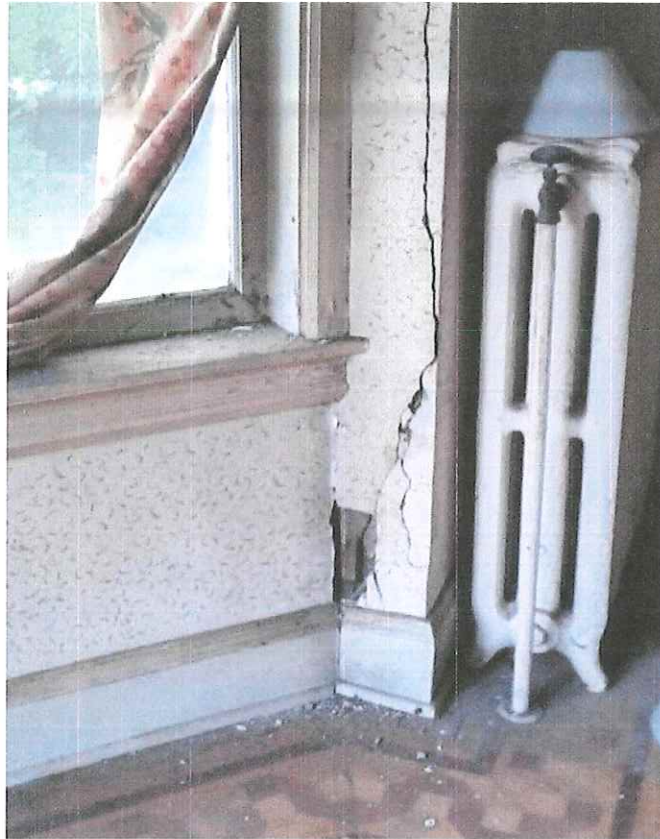
Photograph #7 – Interior first floor wall
