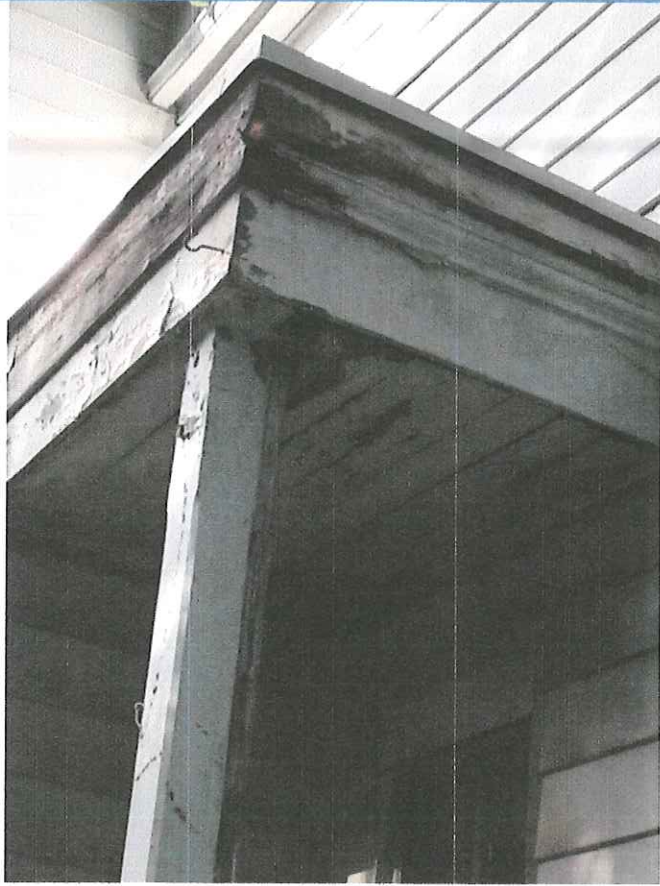
Photograph #5 – Porch roof eave
