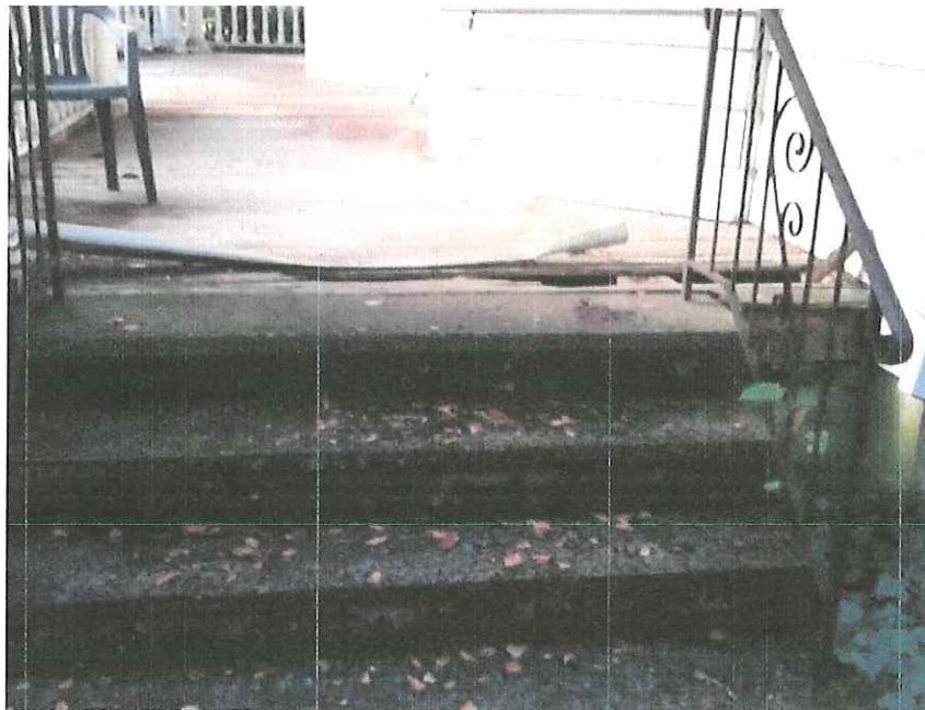
Photograph #3 - Porch floor and supporting columns
