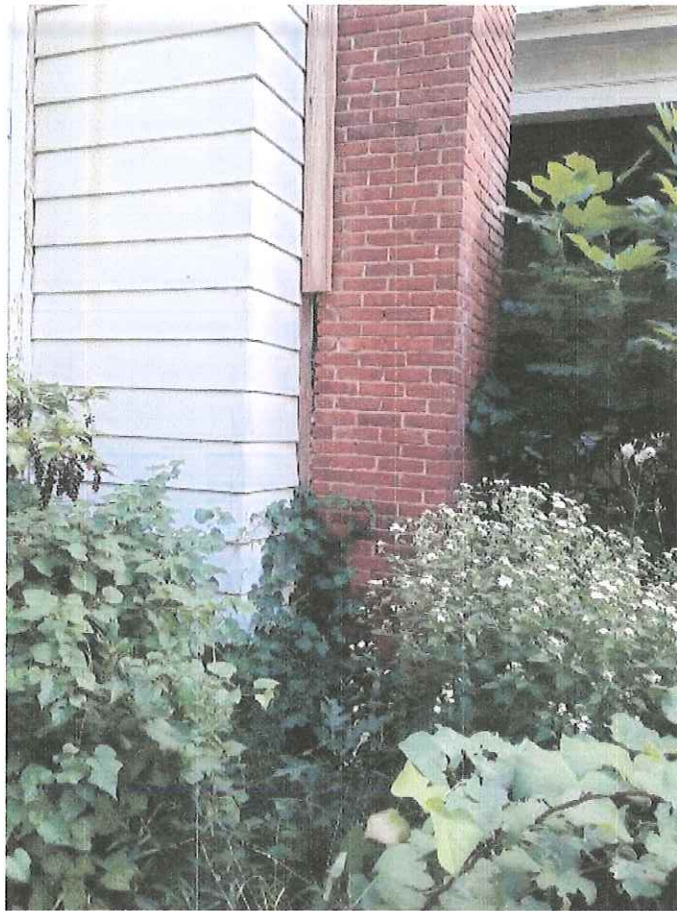
Photograph #17 – Chimney on left side of house
