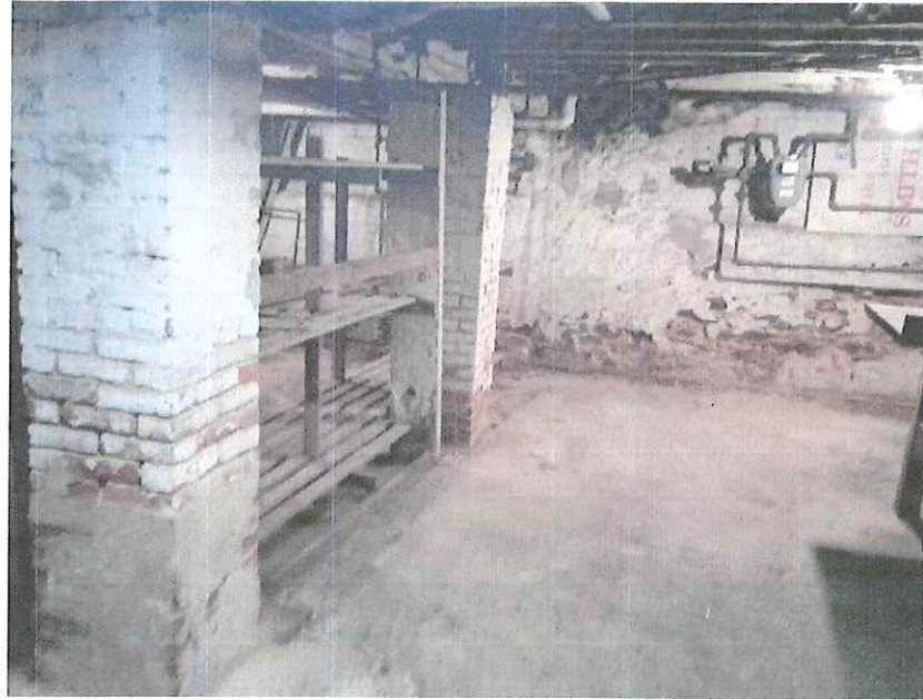
Photograph #1 - Basement walls
